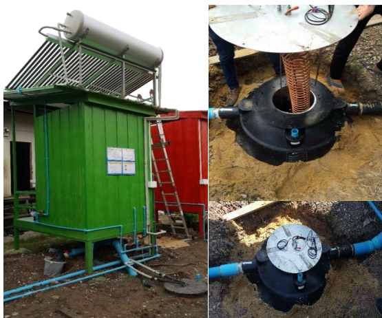
Fig. 4 Field testing of solar septic tank at Santavee factory.
